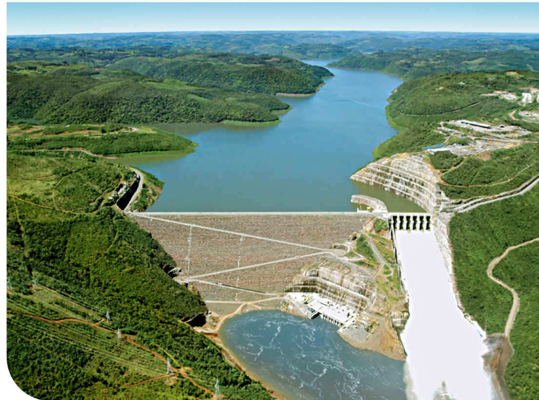
CPFL Geração hydroelectric plant
