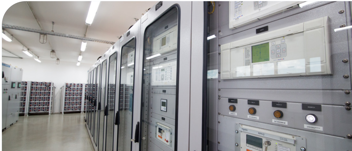
Installation of CPFL Piracicaba
