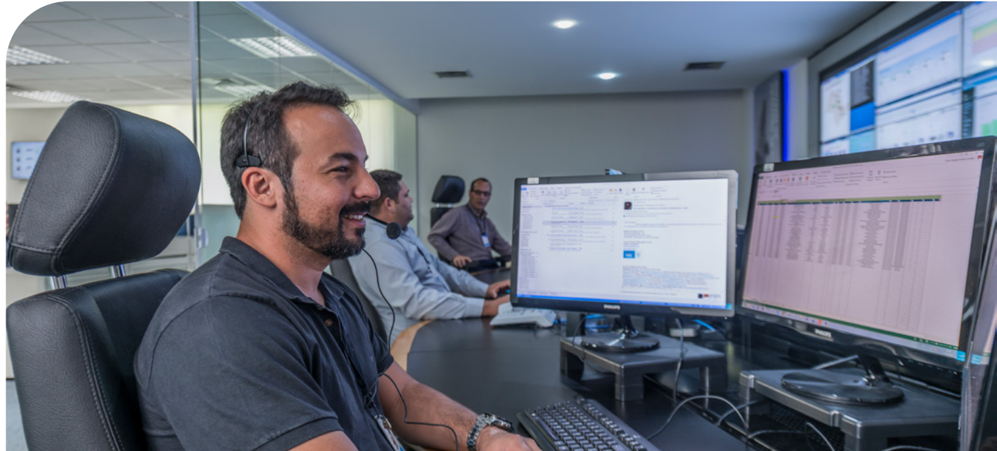
Telecom Operations Center in Campinas (SP)
